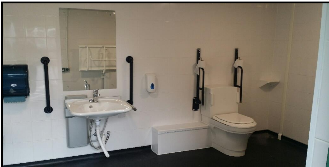
After photo of completed project Tenby Pembrokeshire
