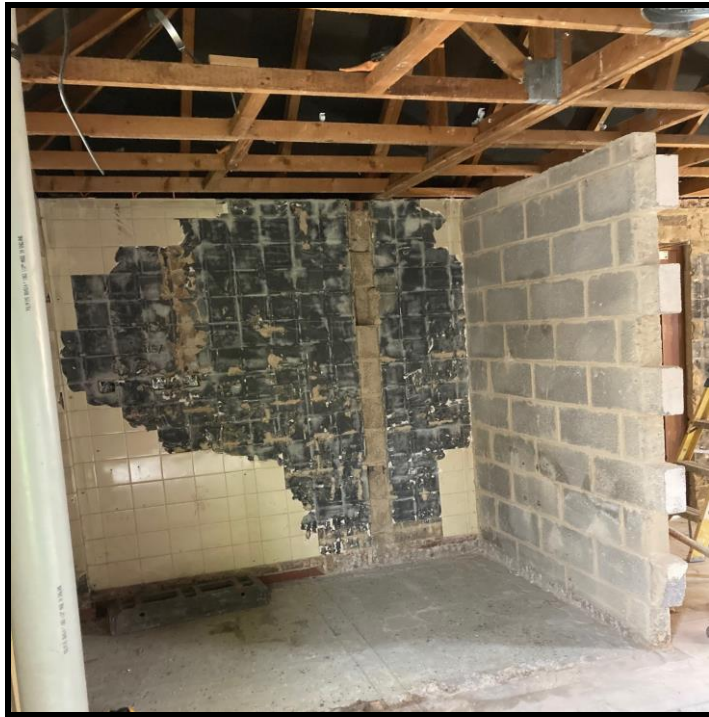
Photo of room at start of recent Changing Places project in Banbury, Oxfordshire
